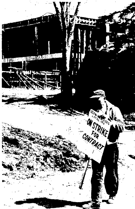
PICKETING STILL continues at the construction site of the new Fred S. Berry dormitory on the Wayne State campus. Picketing by the Ironworkers Union has halted work by all skilled crafts on the project under contract to the Chris Hansen Construction Co., Sioux City.
